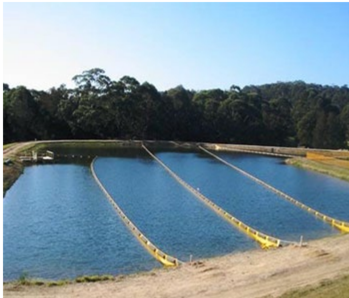
FIGURE 4 INSTALLED BAFFLES IN A POND
